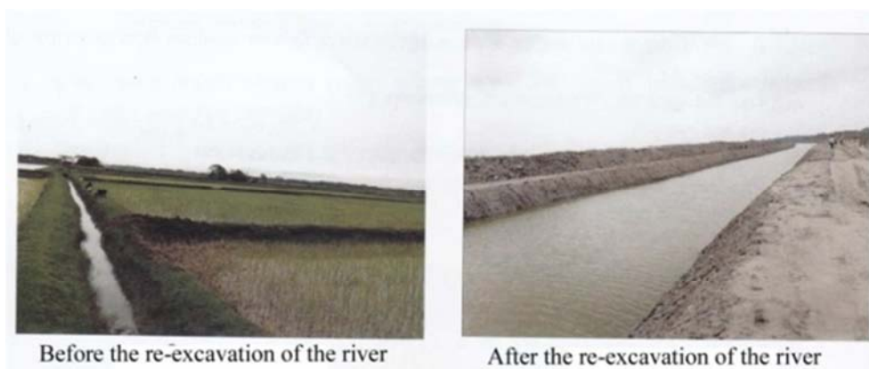
Figure 8. Re-excavation of the River.
